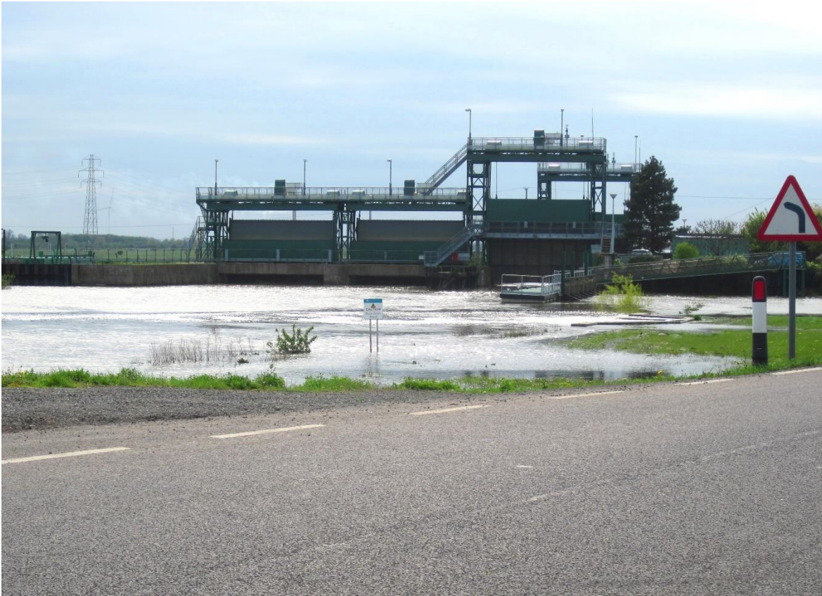
Figure 5-2: Dog in the Doublet sluice during a very high tide. Source: Peterborough City Council
